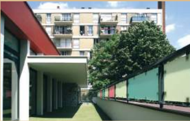
3] Le rez-de-chaussée abrite les unités des “petits” et des “moyens”. The ground floor houses the units for the infants and younger children.
