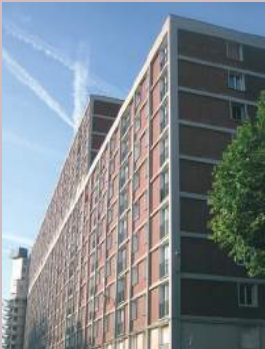
Immeuble Gagarine le long des voies SNCF. The Gagarine building alongside the railway lines.
